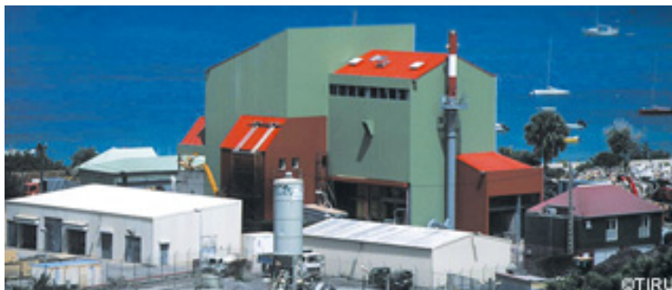
Figure 24 WTE-Desalination Plant of St. Barth
