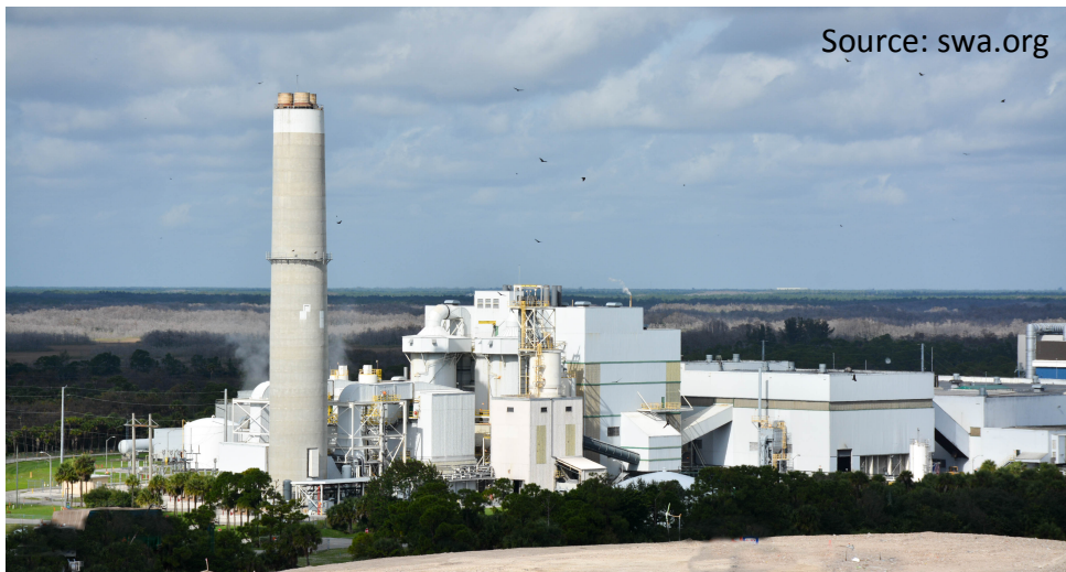
Figure 13 Opened in 1989, the Palm Beach Renewable Energy Facility 1 is an example of waste to energy facility in the United States.
