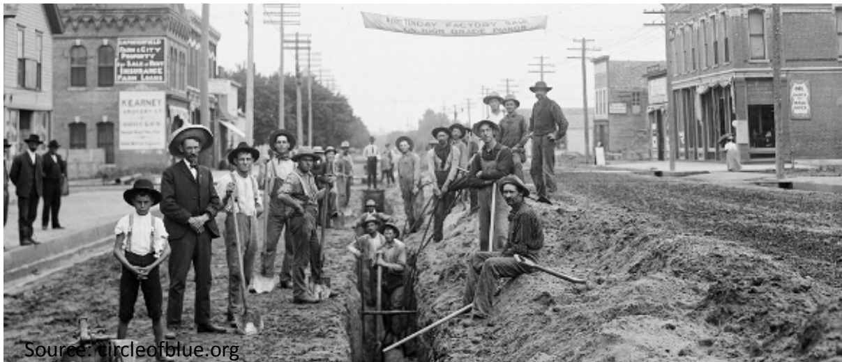
Figure 10 In the late 1800s, public works in America began. The figure above shows , in 1889, the town of Kearny, Nebraska installing sewer pipes for the town.
