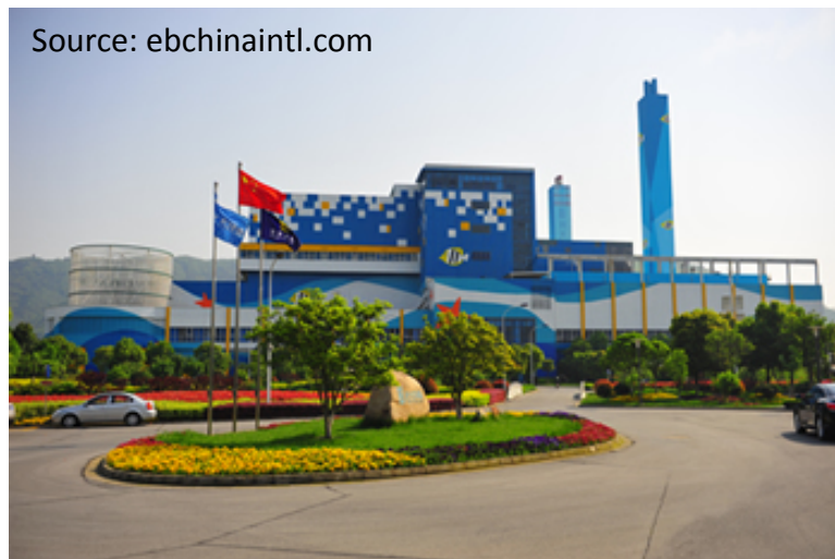
Figure 5 MSW incineration plant, owned by China Everbright International Limited, is located in Suzhou, China.
